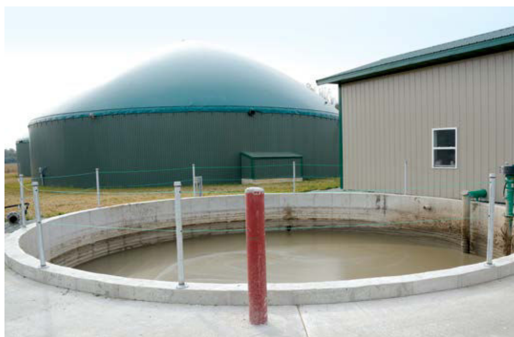
Cow manure is piped to a mixing tank (foreground) that empties into two anaerobic digesters (background).
